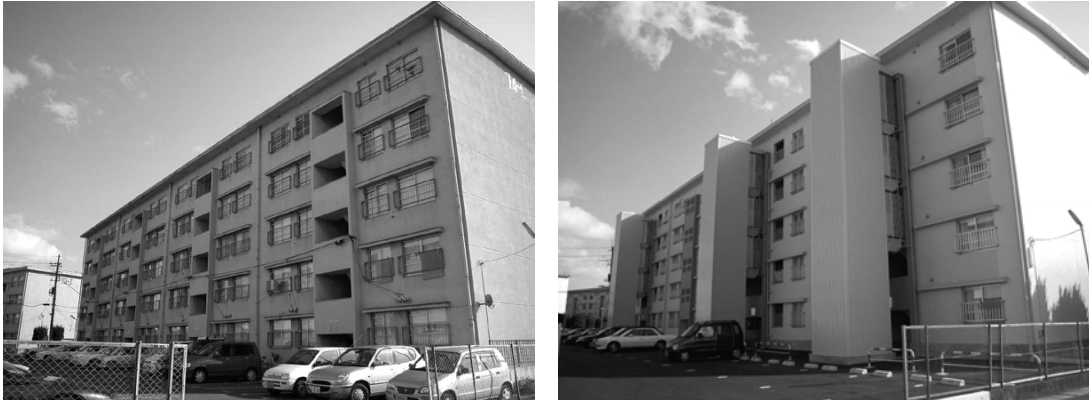
Figure 5 Building Before and After Elevator Towers Addition
