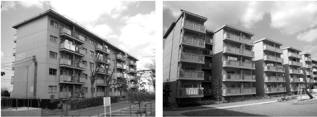
Figure 1 Building Before and After Extension
