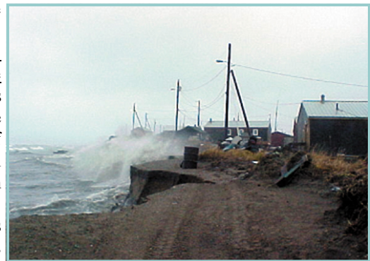
Shishmaref's eroding coastline
